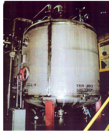
Approx. Dimensions: 8' dia. X 10' high, 700 gpm
